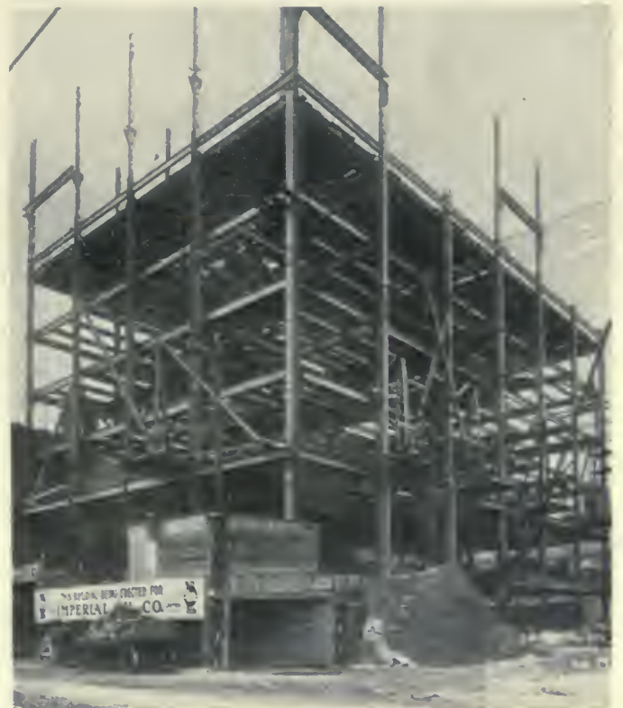
Steel erection, March 21, 1916.
